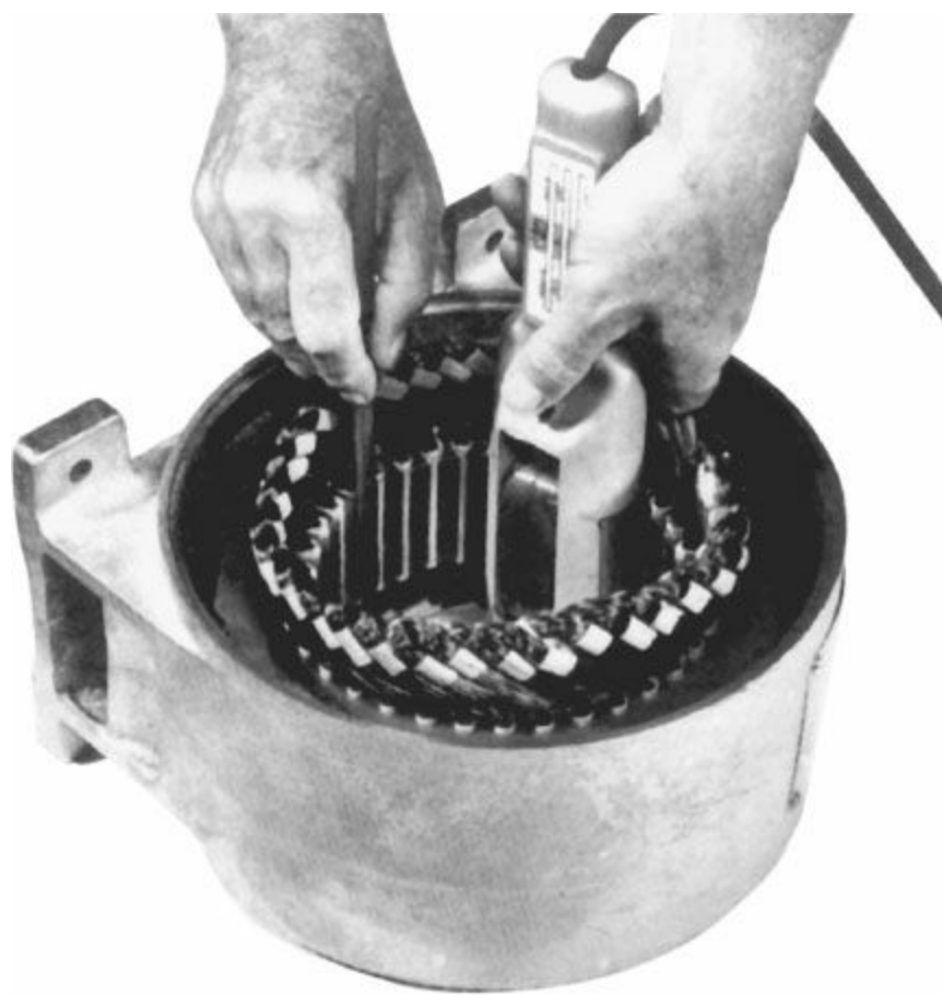
FIGURE 3.30 Checking a stator for a shorted coil by using an internal growler. (Courtesy Crown Industrial Products Co.)
