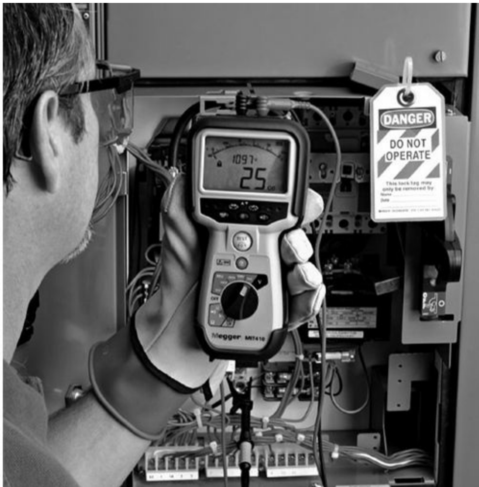
FIGURE 5.25 Panelboard testing using the Megger® insulation resistance tester. (Courtesy Megger®.)
